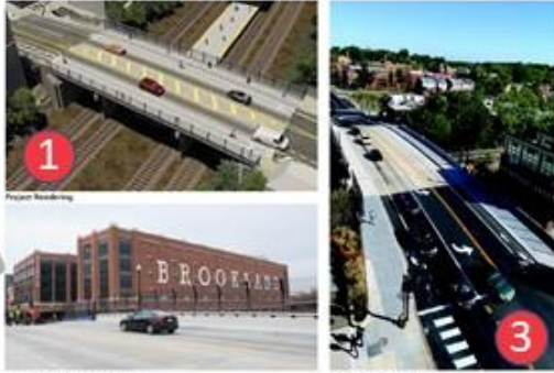
View from Bridge Looking Northwest
